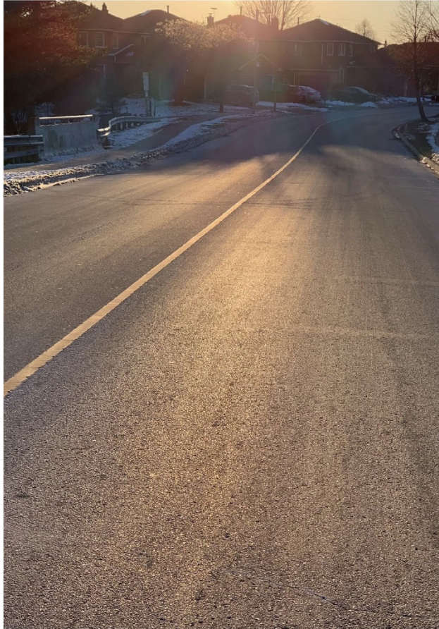
10 lane km of road resurfacing
